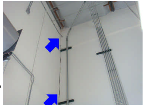
Suspected bent truss strut.
