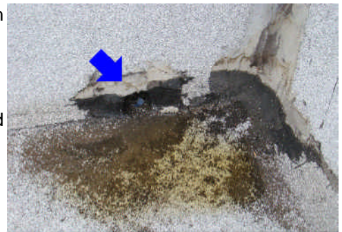
Rear left roof scupper.
