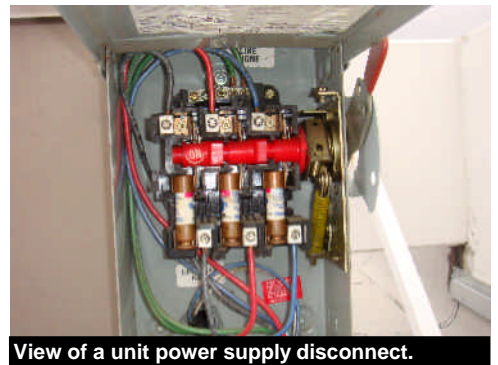
View of a unit power supply disconnect.
