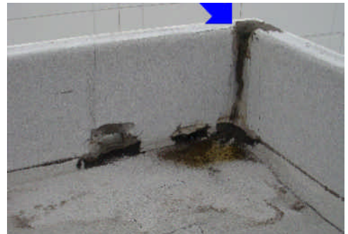
Mastic patching at the rear left corner.
