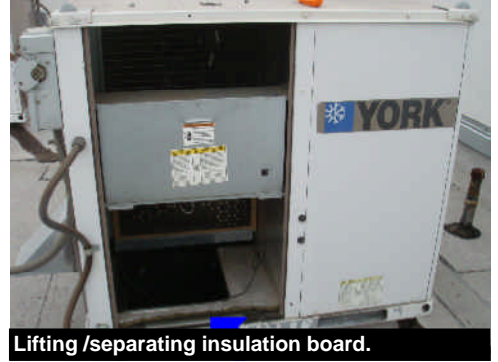
View of a unit power supply disconnect.
